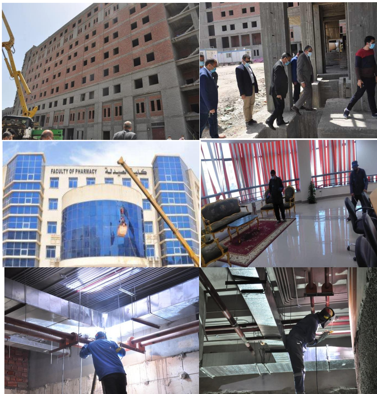
Example of operation and maintenance activities during Covid-19 pandemic
